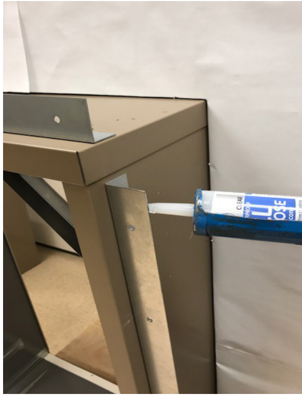
Figure 14: For additional protection against air infiltration during periods of very high winds, fill the clearance space between unit and wall sleeve all around with sealant.
