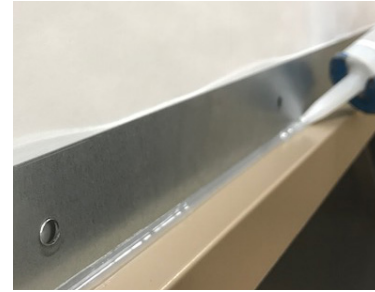
Figure 16: Caulk seal outside joints of wall sleeve before inserting into wall opening.
