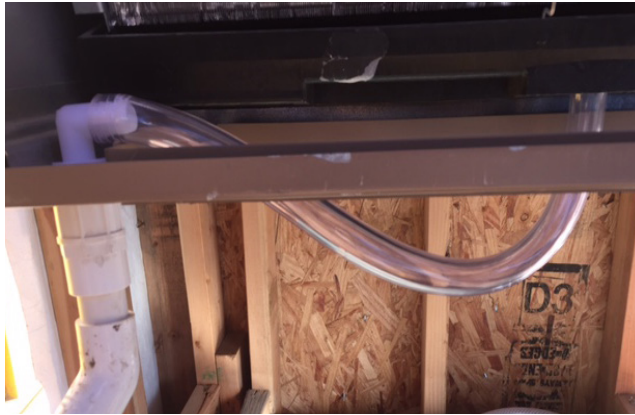
Figure 32: Inside of unit at return-air duct flange, showing sealed condensate tube opening
