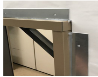
Figure 15: Caulk seal outside joints of wall sleeve before inserting into wall opening
