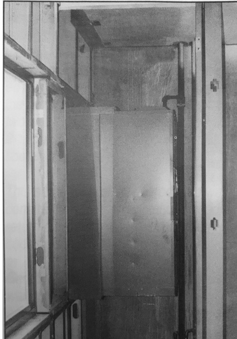
Figure: 27: Wall sleeve fastened to steel 2" x 4" studs with screws fasteners shot through sides of wall sleeve.
