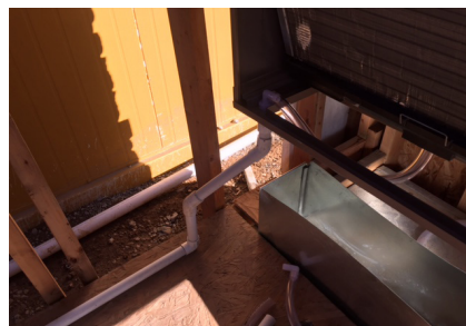
Figure 20: Condensate-tube installed
