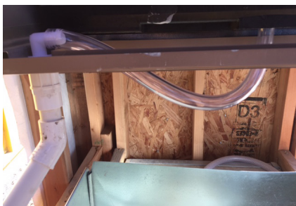
Figure 19: Condensate-tube installed
