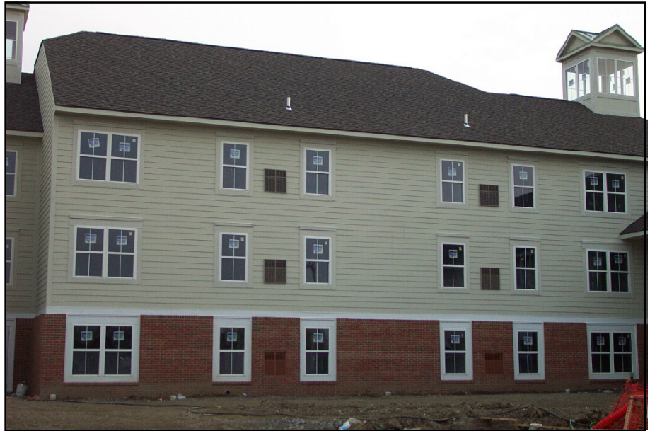
Figure 1 Condominium with Magic-Paks on outside walls
